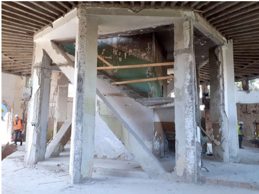
Structural Core – Before Reconstruction
